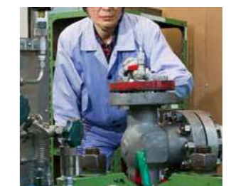
8 Pressure tests Valves are pressurized with air and/or water and operated to verify that they satisfy the quality requirement.
