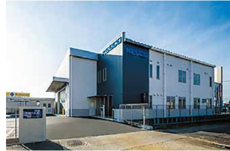
Nagoya Service Center
