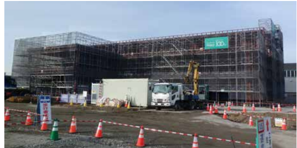
Ongoing construction of the KITZ Group Innovation Center
