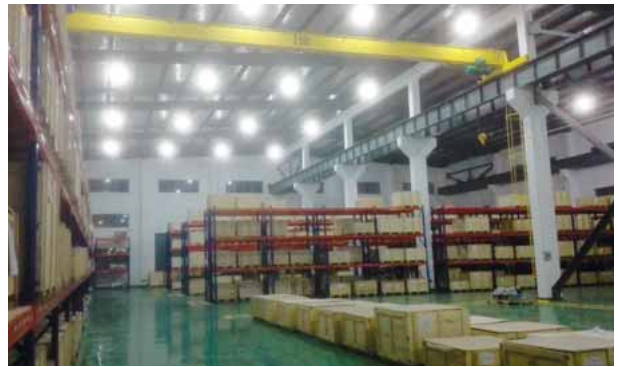
Warehouse at Changshu branch of KITZ Corporation of Shanghai
