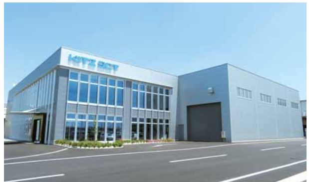
KITZ SCT Corporation dedicated plant for system products
